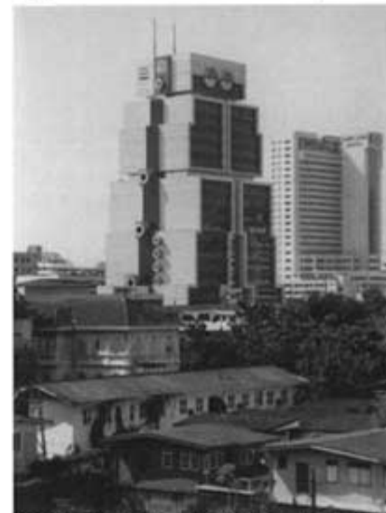
Image: Bank of Asia , Bangkok, Thailand, architect - Sumet Jumsai [photograph by Dave Beynon ]
