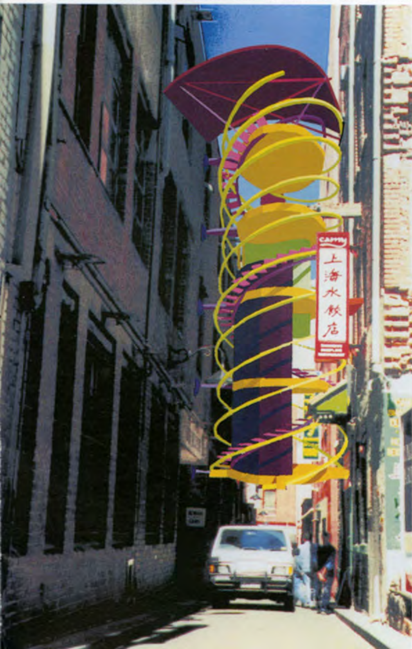
The Slinky House designed by Melbourne architectural firms Also/CAN Pty Ltd and Multiplicity. Winner of Museum Victoria's Home of the Future Competition 1998. Photograph courtesy of Museum Victoria
